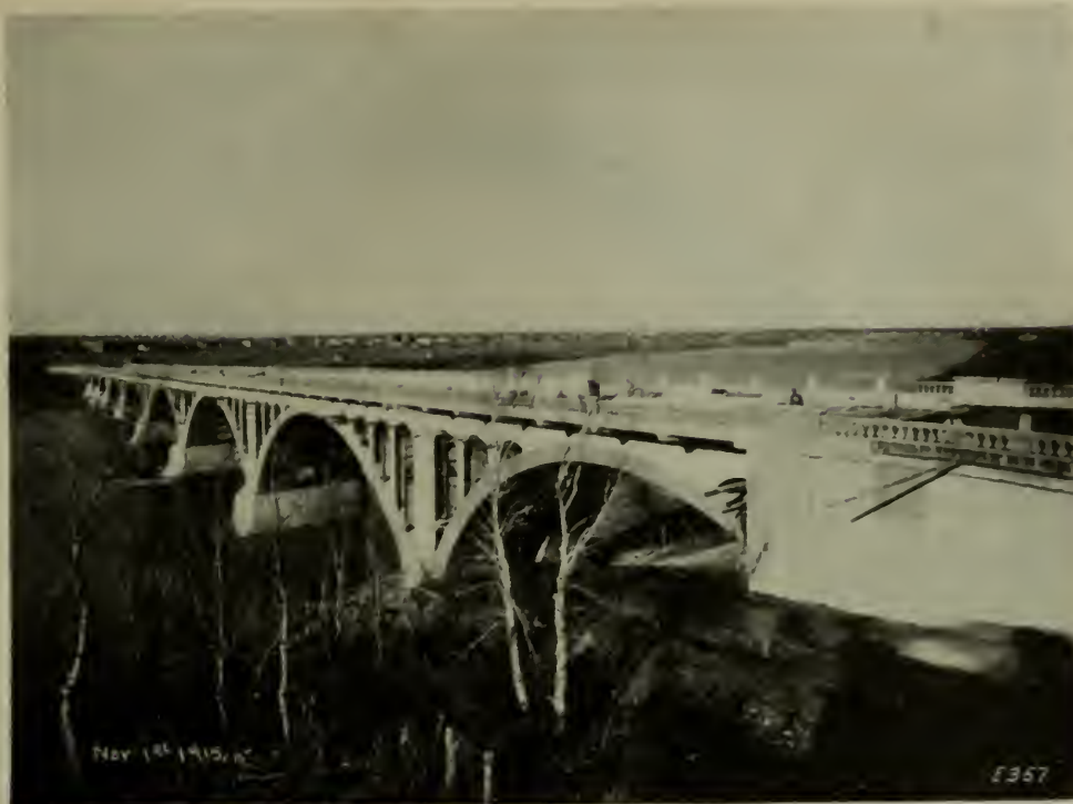
REINFORCED CONCRETE BRIDGE AT SASKATOON.
